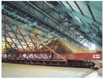
Bridge reclaimer for limestone (cement plant)
